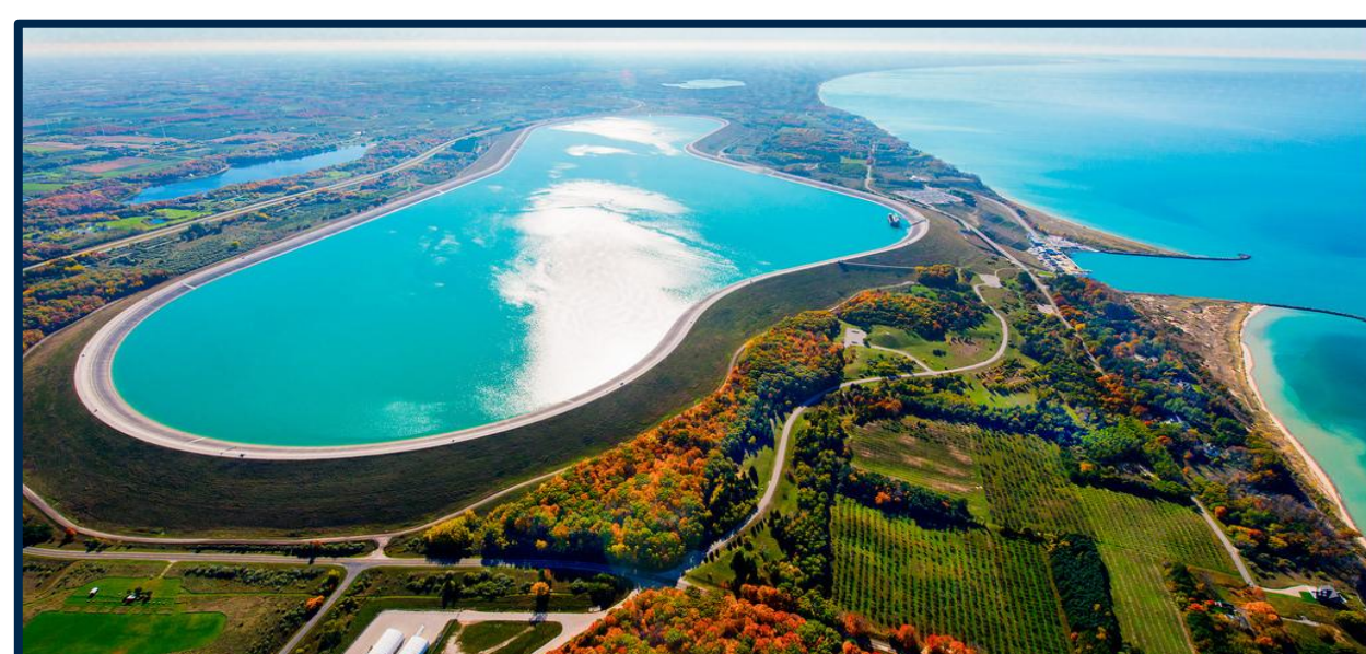
Aerial image of the Ludington Pumped Storage Facility [3].
