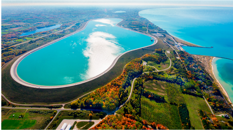
Figure 2.7: Aerial image of the Ludington Pumped Storage Facility. The light blue “lake-type” body of water is the stored water that has been pumped up from the large lake below (on the far right of the image).
